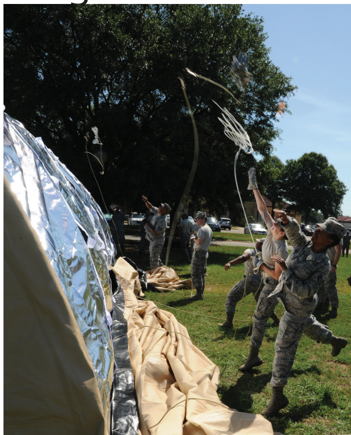
Rope toss: Several members throwing ropes over the Alaskan shelter tent. The ropes were then used to pull the outer canvass into place.
